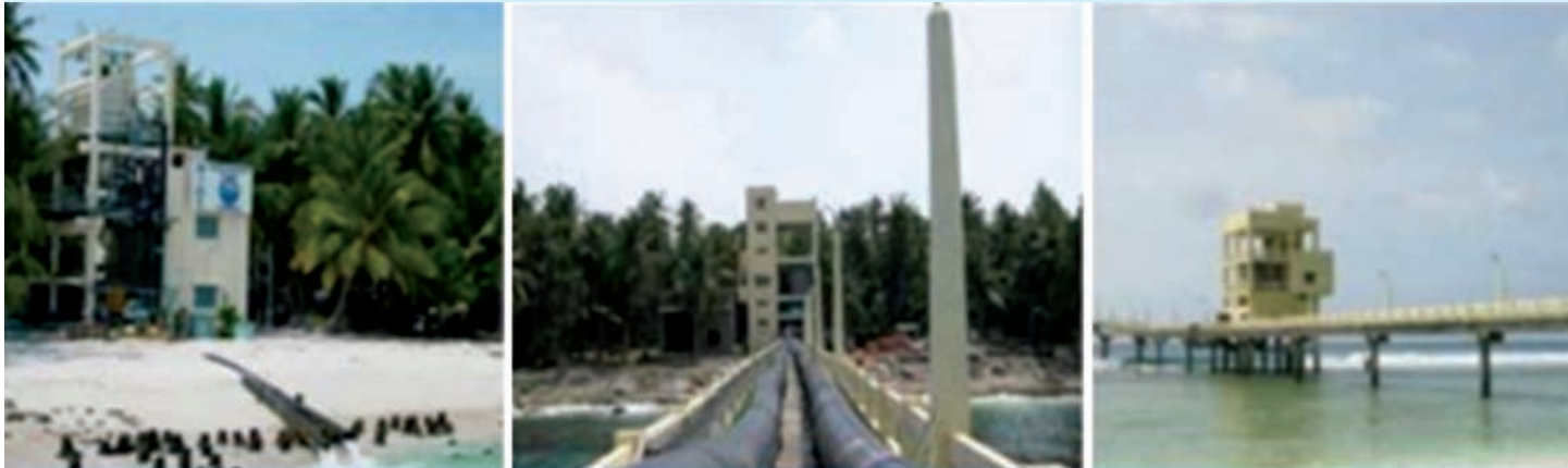
Desalination plant operational in three islands of Lakshadweep
