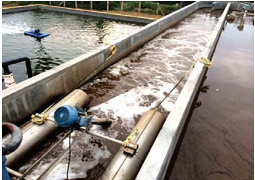
Water Treatment Facility & Waste Water Treatment Plant at Thirupattur, Vellore, Tamil Nadu
